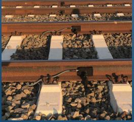
This signal sensing module is attached to the rail for sensing the acoustic signals generated by the RAG100 unit. It first detects and processes the detected acoustic signal and communicates with the track-side electronic board for additional signal processing and communication.
